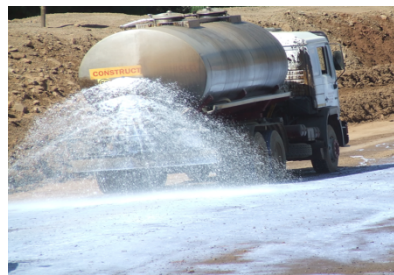
ii. Spraying SoilTech Mk. III
