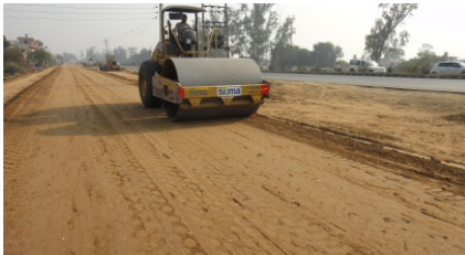
iv. Rolling & compaction
