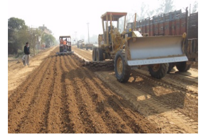
iii. Mixing & grading
