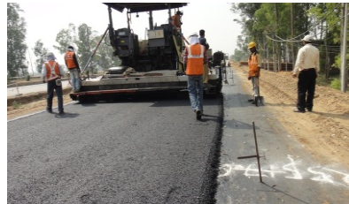
v. Laying Wearing Course
